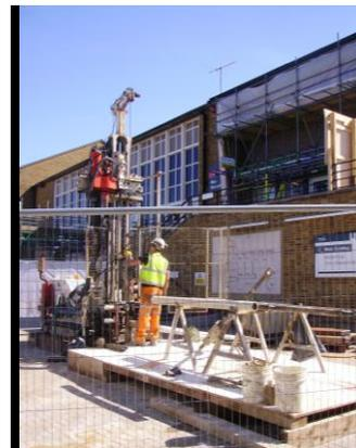
Fig 2. Example of borehole rig at Prince Edward Hall
