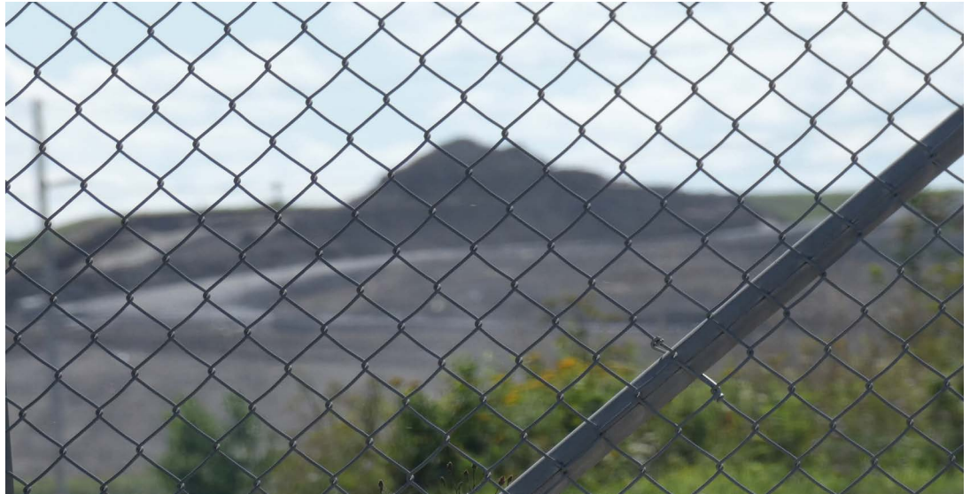
Fig. 1 Digital Photograph. Landfill (Alcoa, Massena, NY), 2020. Photo courtesy Maria Taliano. This image is from an active landfill.
