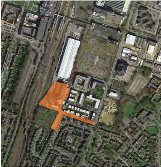
Bio Park Disposal 2020/2024
