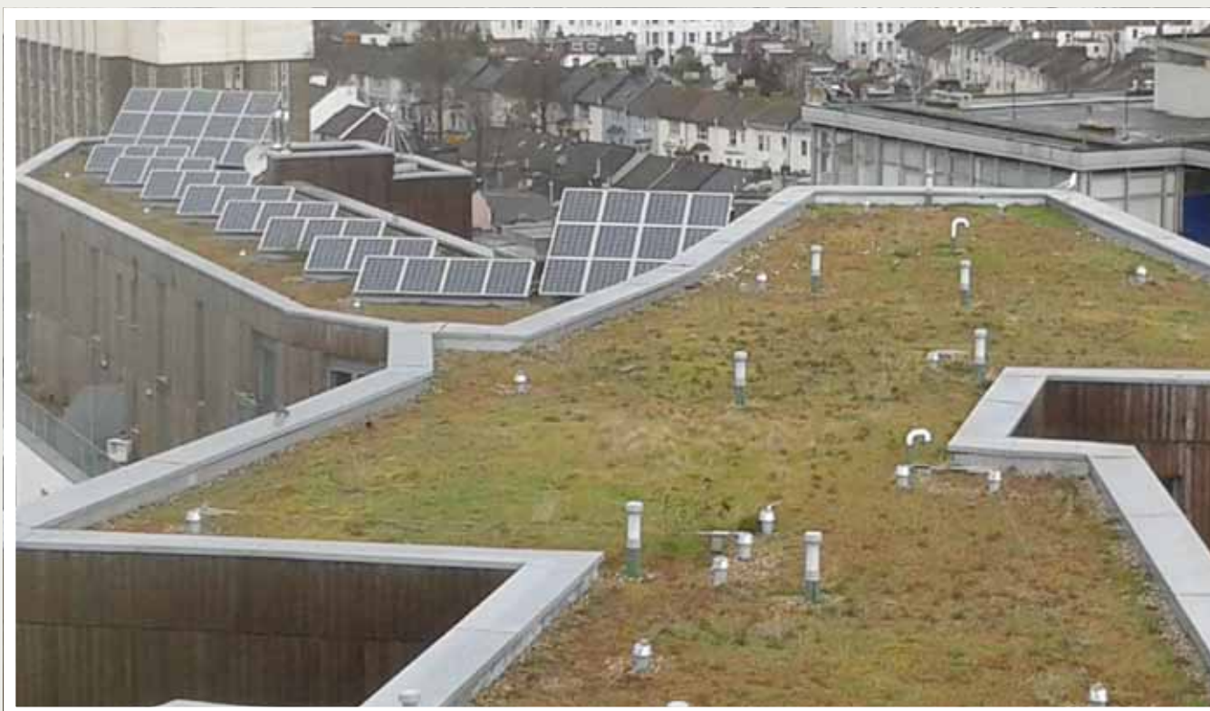
Figure 16. Solar panels and green roofs at One Brighton
