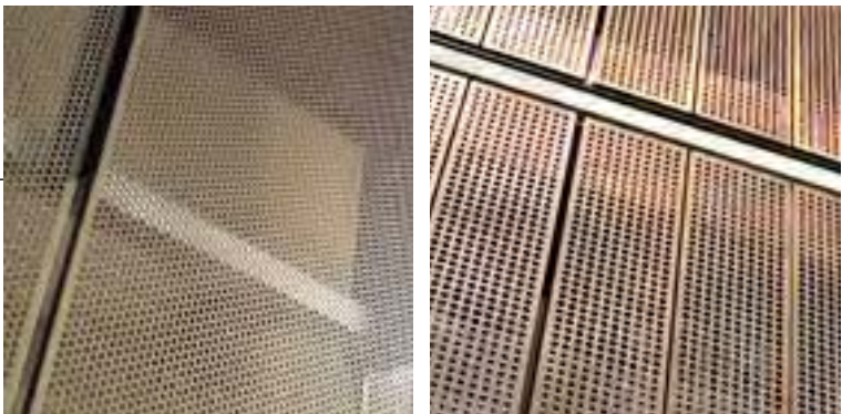
Perforated metal cladding to solar shading/ spandrel panel
