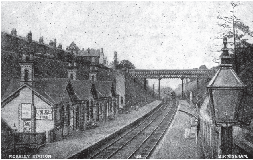
Figure 2.2. Moseley station, late nineteenth century. PCRC.
