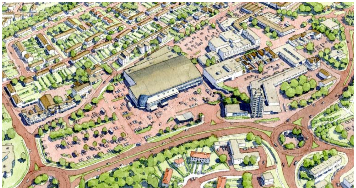
A greyfield site, with an enclosed shopping centre and multiple car parks. In this case, Hatfield New Town Centre as existing
