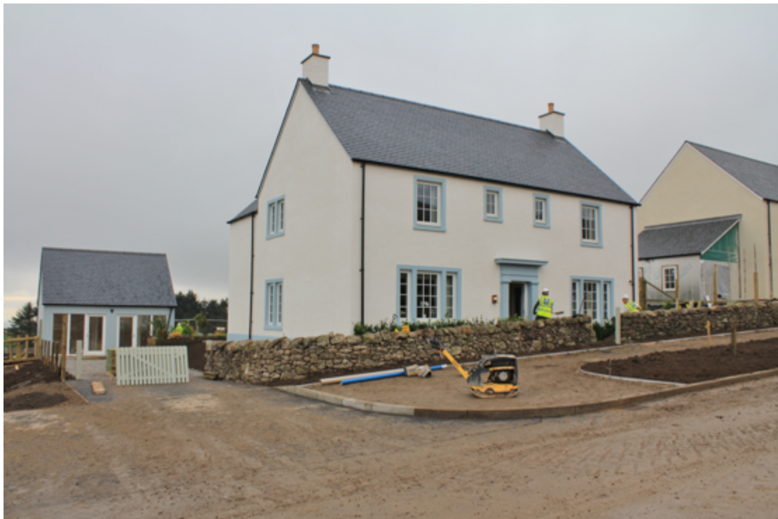
Example of new house construction in Chapelton Source: Brooks Murray Architects
