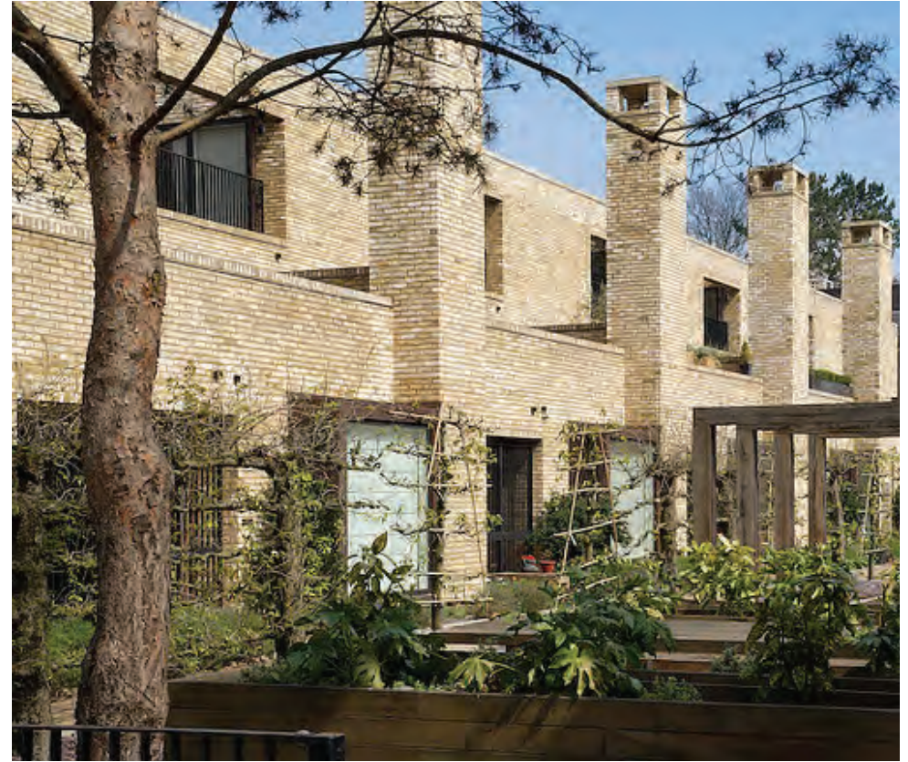
Figure 6: New housing at Accordia, Cambridge (Source: Wikicommons)
