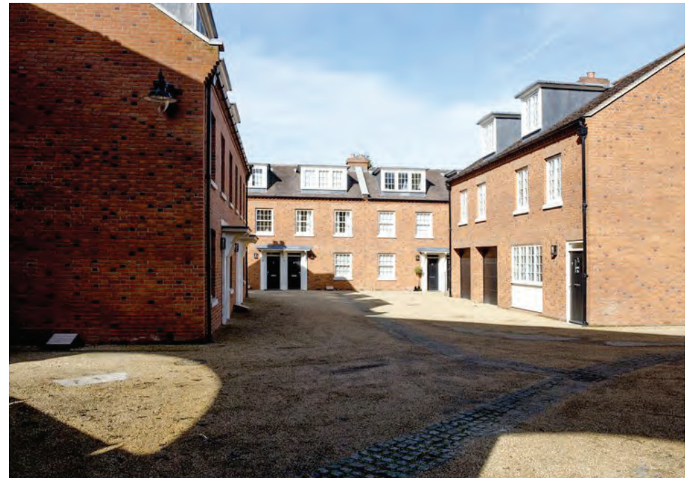
Figure 8: Small infill redevelopment in Old Hatfield (Source: Gascoyne Cecil)
